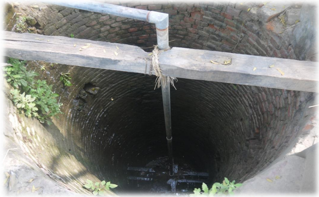
Figure 18 : Boring in a former well
